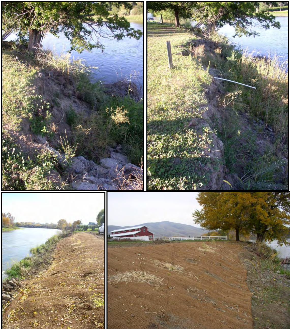
Riparian stabilization at Crawford Property. Prior to restoration (top), after restoration (bottom).
